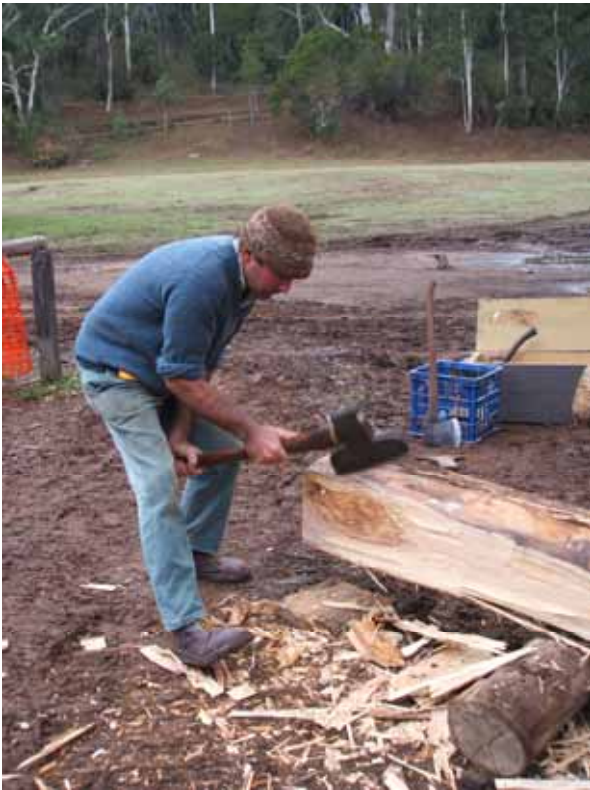
Timber post preparation by James Finlay. Photo: Courtesy of Ken Birch
