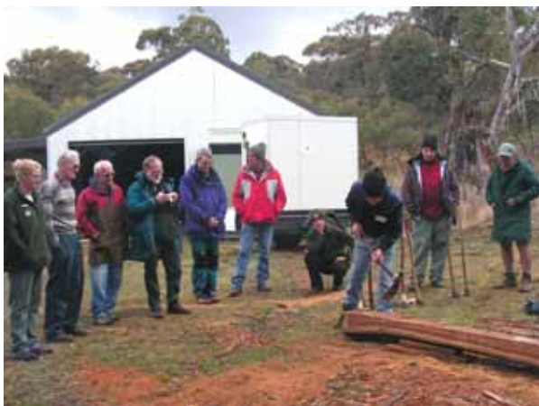
Some adze work on timber post preparation. Photo: Courtesy of Fiona Magnussen.
