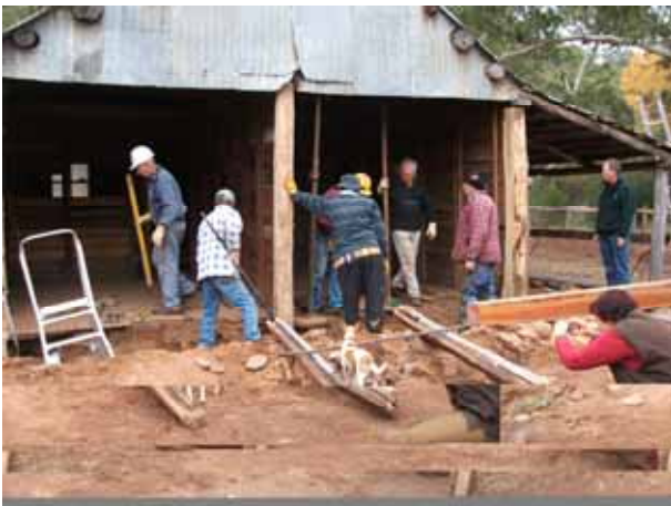
Removing floor & securing roof. Photo: Courtesy of Ken Birch
